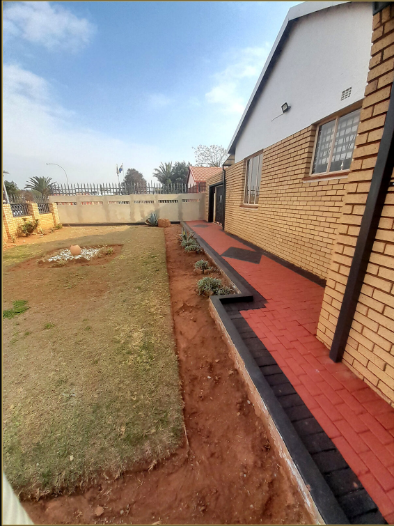
Red paving laid along the side of the house
