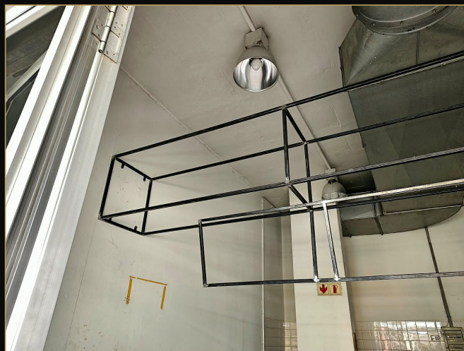
Steel bulkhead frame
