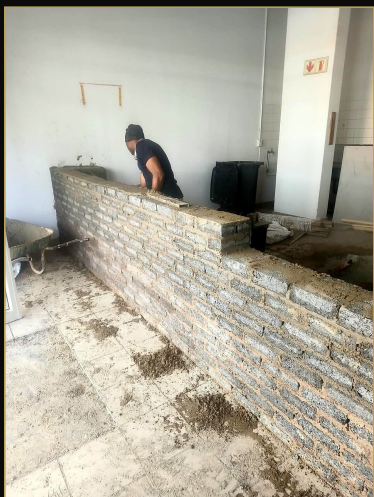
Counter brickwork going up
