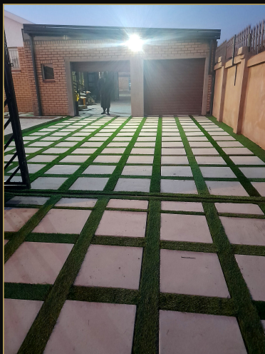
Driveway slabs and grass strips
