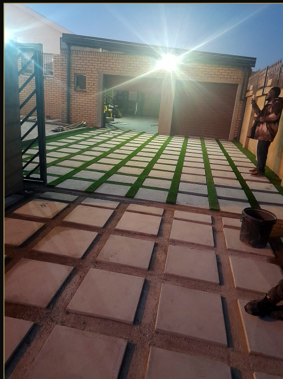
Driveway slabs and grass strips going in
